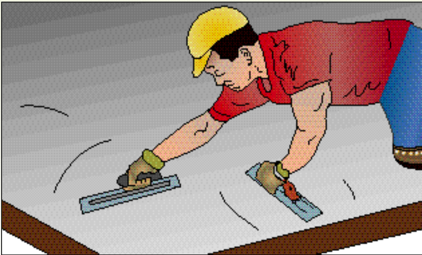
Gloves are a must when you are finishing fresh concrete.
